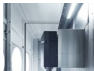
LED lighting in the working area.
