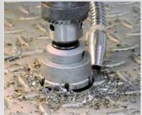
Drilling in checker sheet
